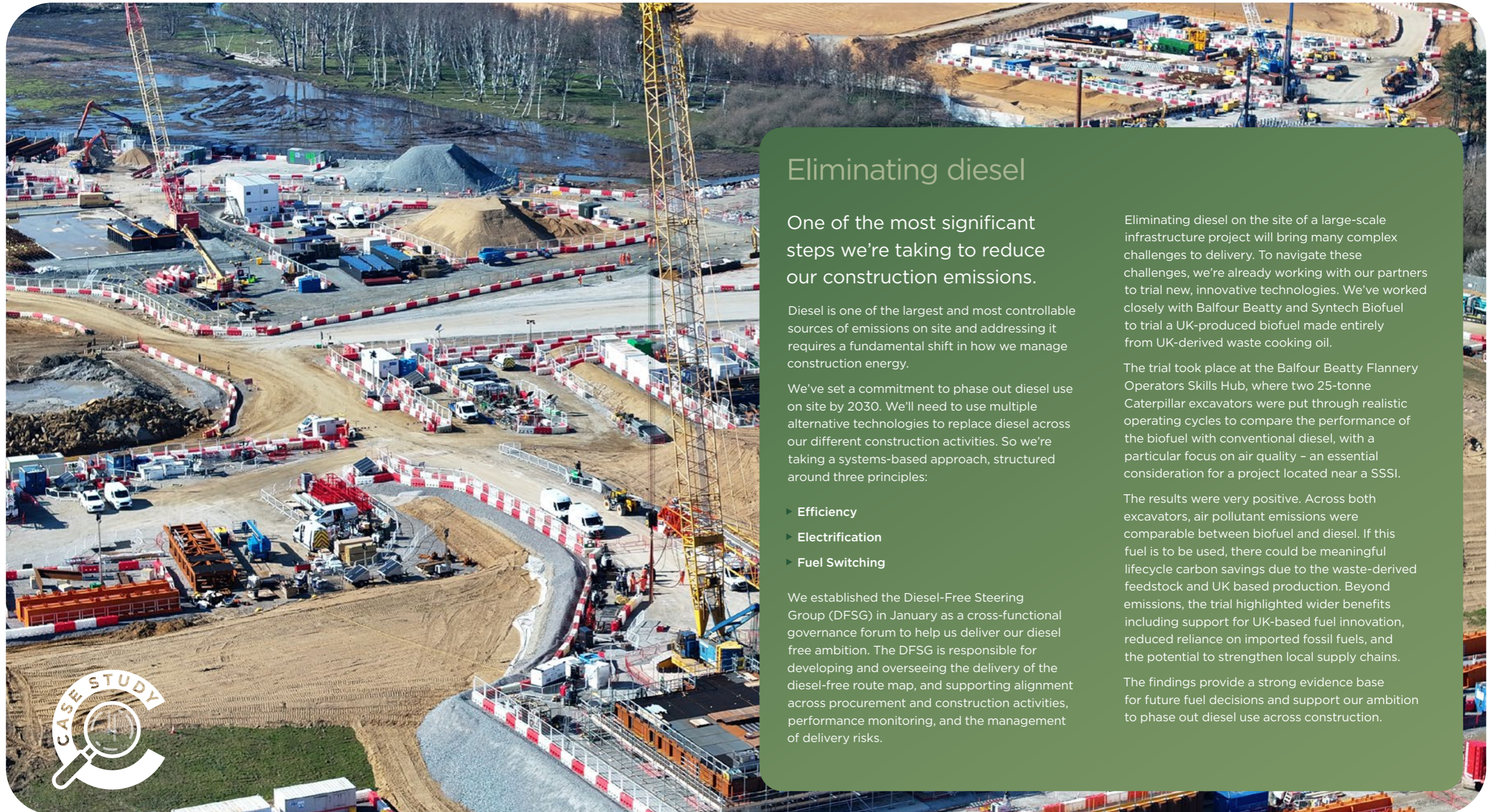
Image: The Main Construction Area.
