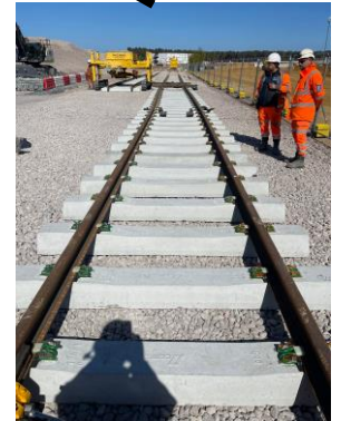
TCA – last panel installed 21/4
