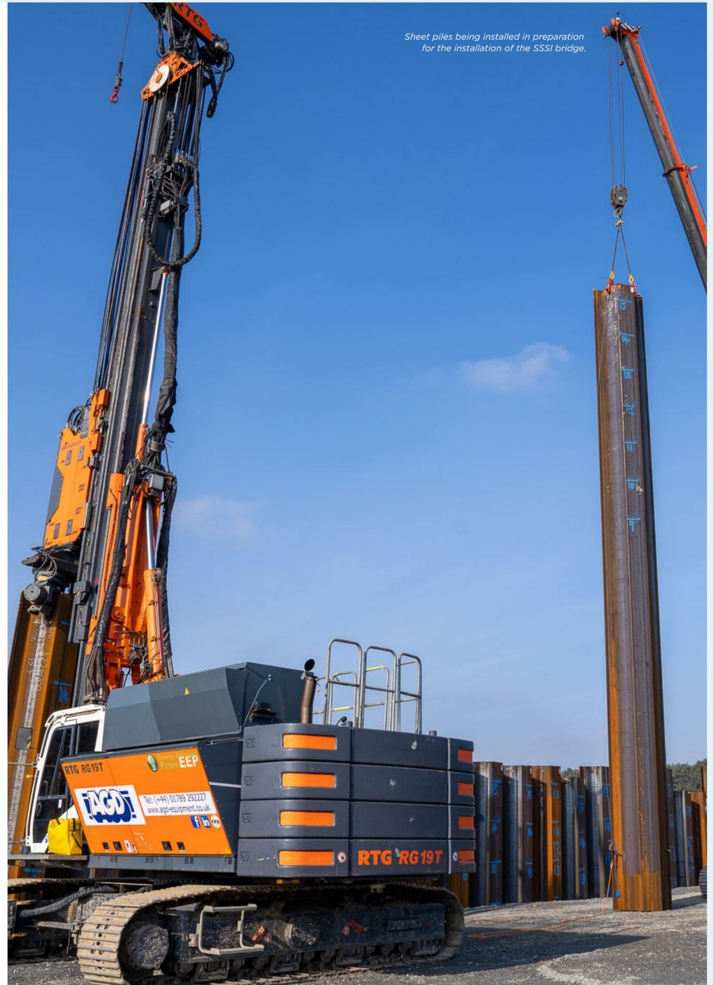
Sheet piles being installed in preparation for the installation of the SSSI bridge.
