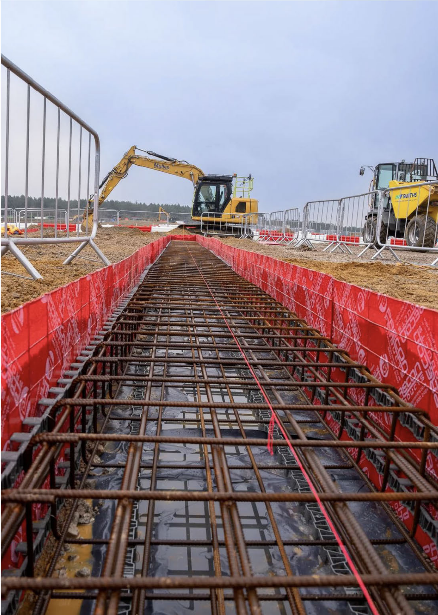
Pictured right are foundations being laid on the Temporary Construction Area at the Sizewell C site in Suffolk.
