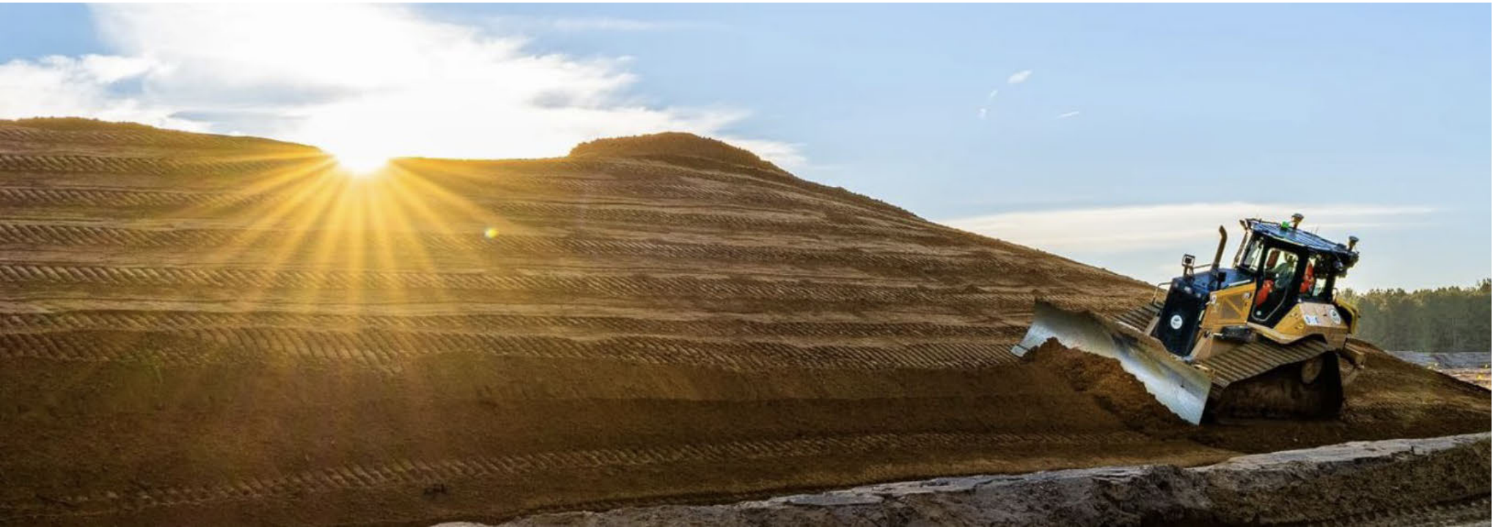
Pictured below is a dozer moving earth on the Temporary Construction Area in November 2024.
