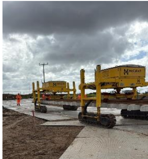
Plain line Track Panels Delivery
